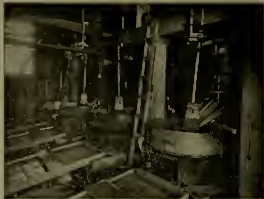
Interior of a Four Kinkhead Quartz Mill Plant equal to 20 stamps, supplying four 6-foot concentrators in operation at Virginia City, Nevada. Capacity, 40 to 50 tons every twenty-four hours through 40-mesh screen.
