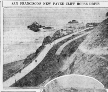
SAN FRANCISCO'S NEW PAVED CLIFF HOUSE DRIVE. NEW HIGHWAY REPLACES OLD CLIFF DRIVE.
