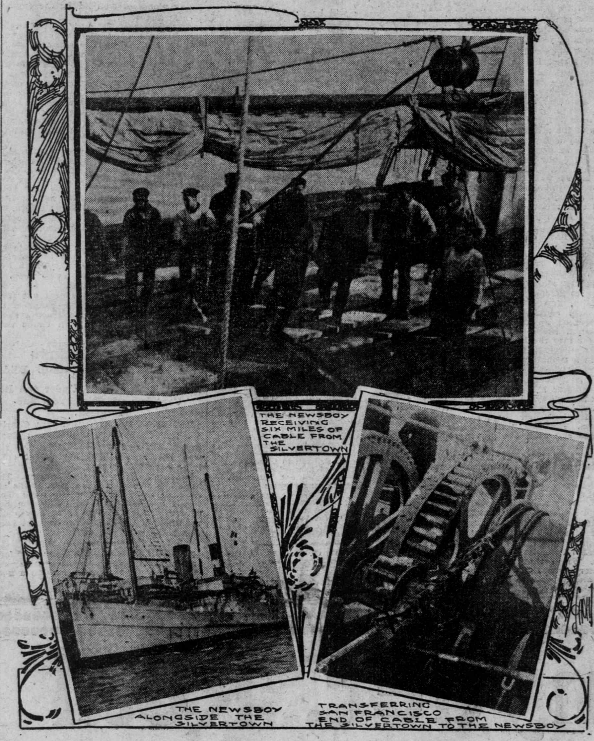
PHOTOGRAPHS SHOWING PREPARATIONS THAT WERE BEING MADE YESTERDAY FOR A SECOND ATTEMPT TO LAND THE SHORE END OF THE GREAT PACIFIC CABLE ON THE OCEAN BEACH BELOW THE CLIFF HOUSE.
