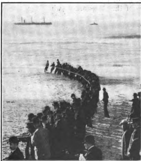
WEIDNER, PHOTO FIRST ATTEMPT TO HAUL IN THE CABLE—THE CROWD PICKING UP THE HAWSER SLACK
