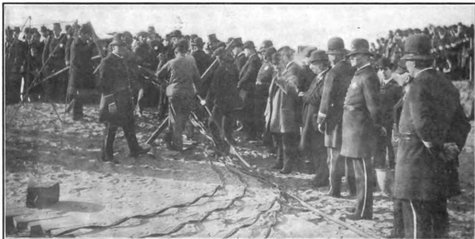
DANA. PHOTO REMOVING COVERING OF SEA END OF CABLE, BEFORE SPLICING
