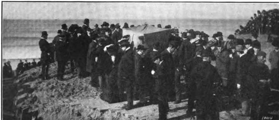
TABER, PHOTO CONNECTING JOINTS OF INNER COILS OF THE CABLE—THIS IS DONE UNDER COVER IN ORDER TO KEEP OUT ALL DUST
