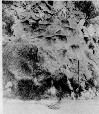
Across the street from the Cliff House, workers continue their war on a mass of base rocks. The rocks, made of a concrete like substance, were built in 1925 and of late have been rapidly deteriorating. The demolition will take about two or three weeks, according to the National Park Service, which is in charge of the operation.
